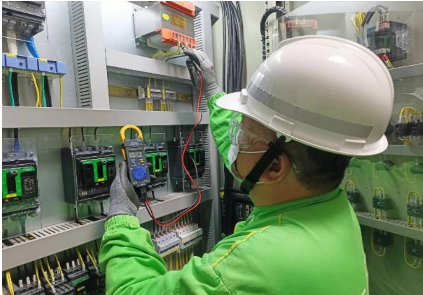
Power Distribution Panel Maintenance
